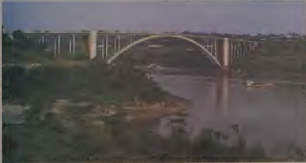
Bridge over the Alto Paraná River between Ciudad del Este, Paraguay, and Foz do Iguazú, Braz.
